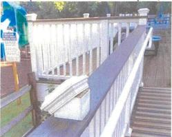
All sharp edges formed by cutting the trex material shall be eased to a 1/8" min 6. radius.
